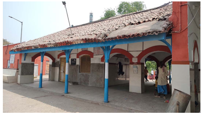
Figure 11 : Kursela Railway Station, Muradpur Source: Primary survey by AH Division, INTACH Team
