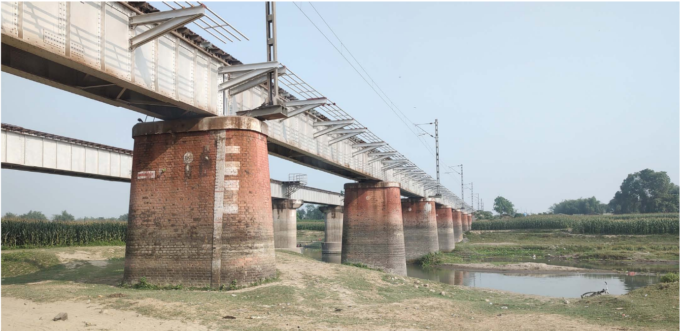
Figure 1 : Old Railway Bridge at Barari.
