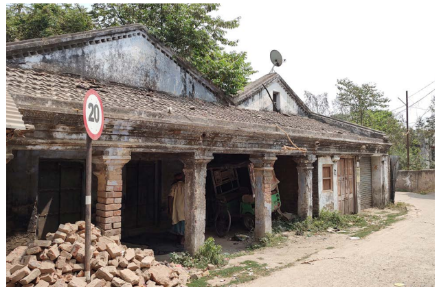
Figure 21 : Abandoned Residence in Ayodhyaganj Bazar, Kursela Source: Primary survey by AH Division, INTACH Team
