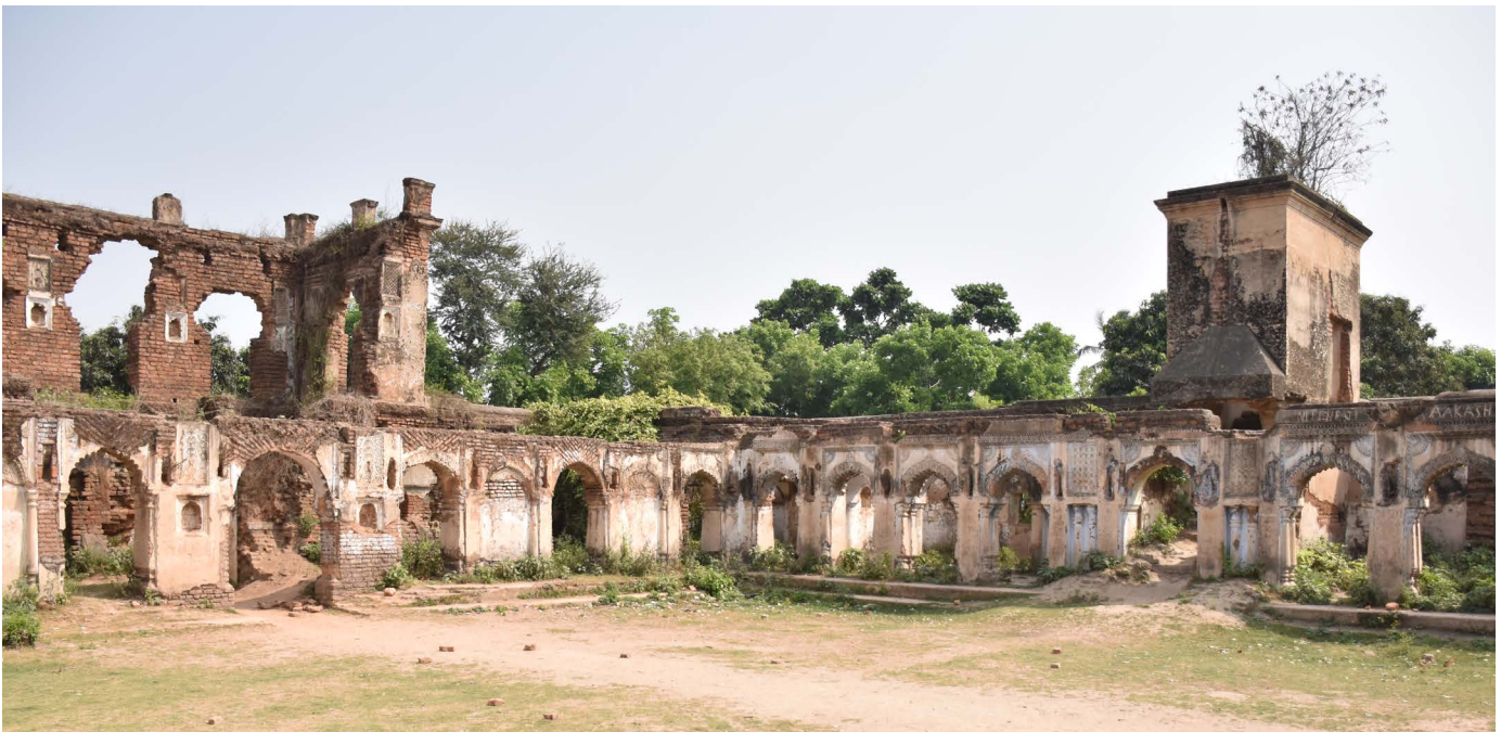
Figure 7 : Bairam Singh ki Kothi, overlooking Burhi Gandak River. Source: Primary survey by AH Division, INTACH Team
